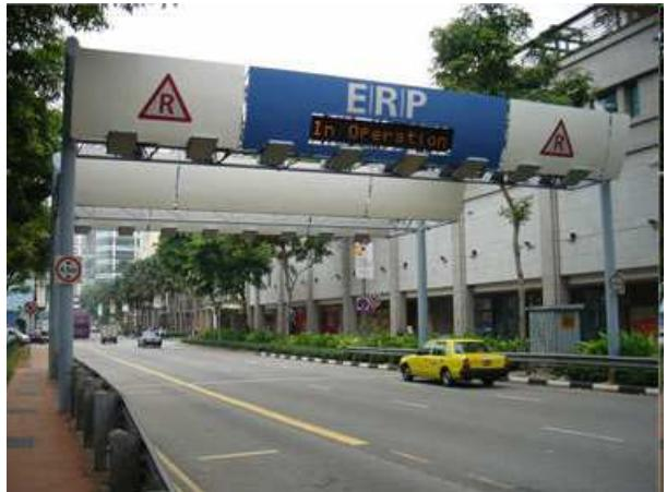
The electronic toll system, set up in Australia, Singapore or in the United Kingdom, allows to automate payments and to reduce bottlenecks by identifying vehicles on which RFID tags are embedded.
